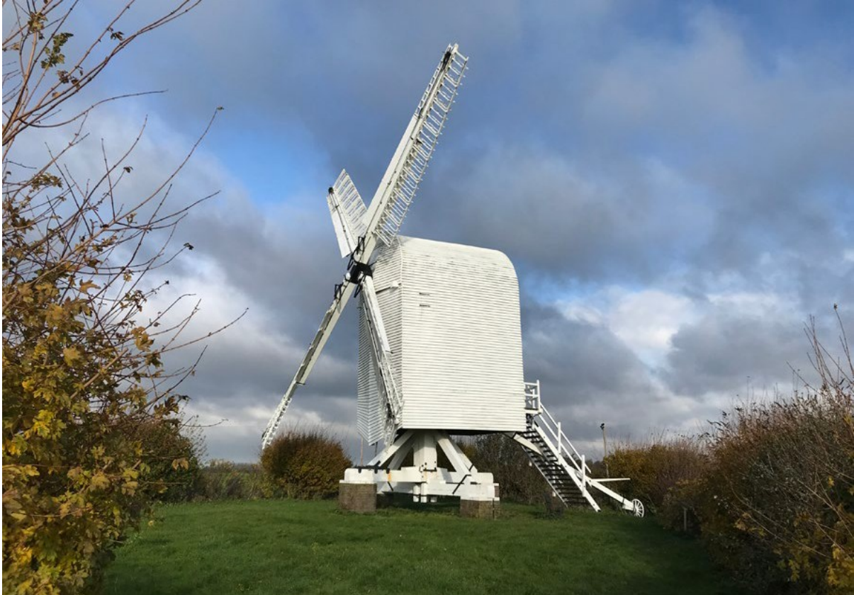
Figure 7 Chillenden mill after restoration.
