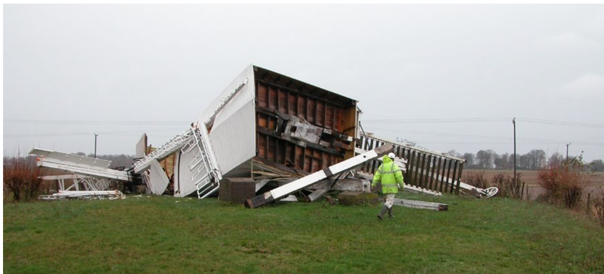
Figure 6 Chillenden windmill, blown down in 2003, now re-built.
